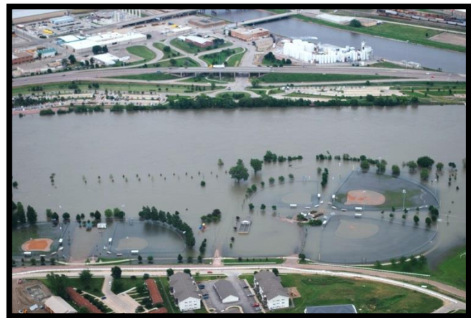
Figure 4. South Sioux City used their floodplain for ballfields that didn't put lives or property at risk
