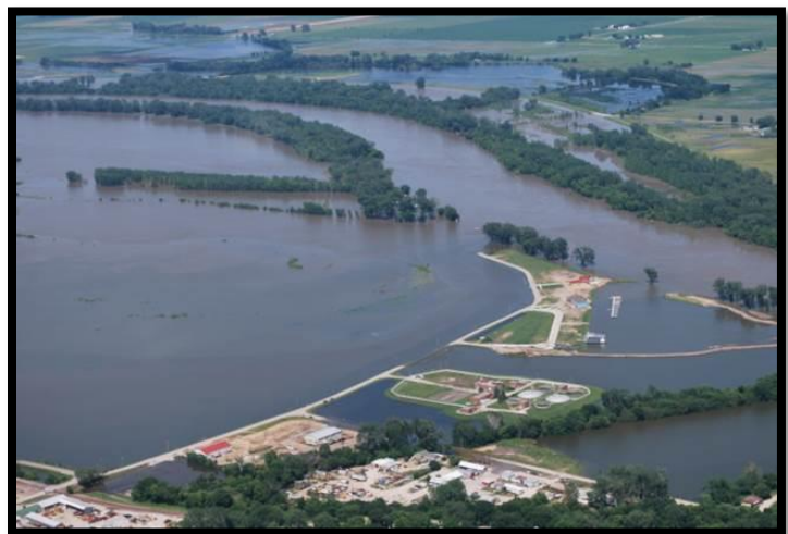
Figure 7. Plattsmouth wastewater treatment plant threatened by Missouri River in 2011
